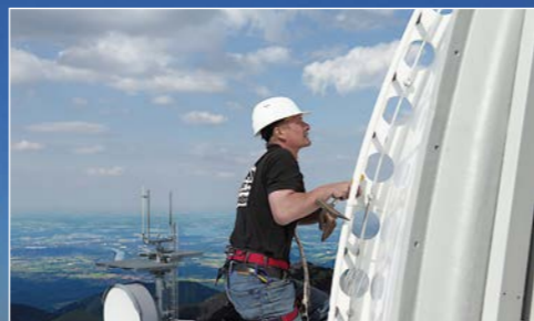
Wendelstein, Germany – mounting of 8.5 m Dome
