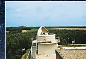
Rocket test ground 5.5m high speed Dome
