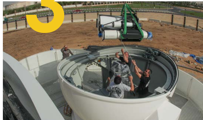
The team inspects all components and installs your observatory.
