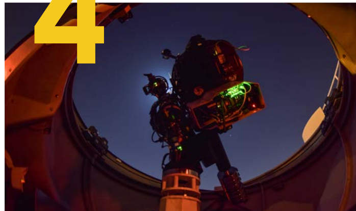
Once installed, the team takes the first astronomical image to ensure functionality and system performance.
